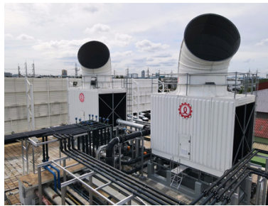
Cooling Tower Installation
