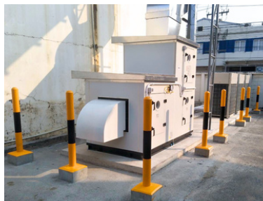
Air Handle Unit Installation
