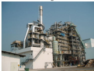
Instrument work installation
