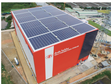
Solar Power Generation
