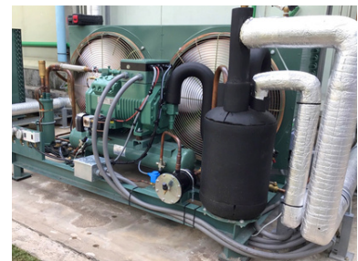
Compressor Unit Installation
