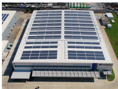
Solar Power Generation
